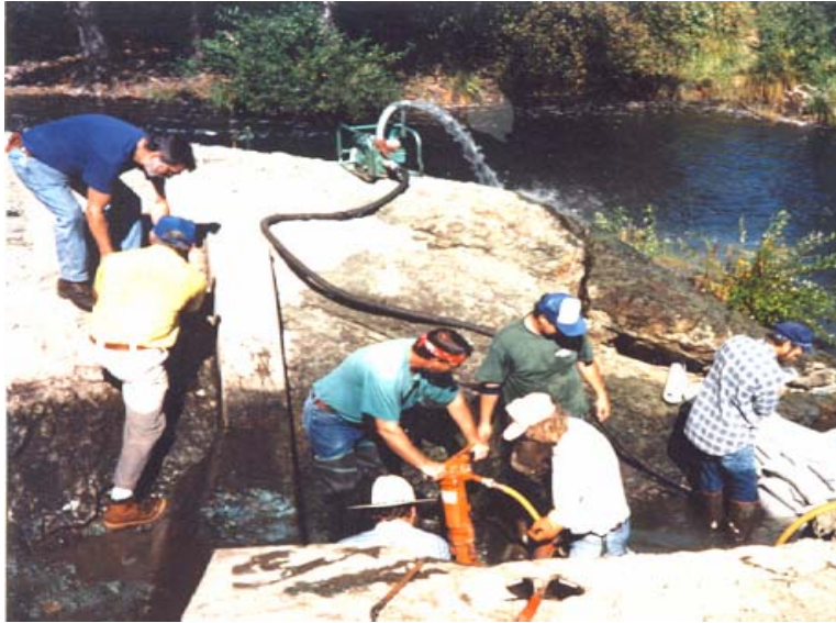
Members of the URWA work to deepen the approach to a fish ladder on Big Butte Creek.
