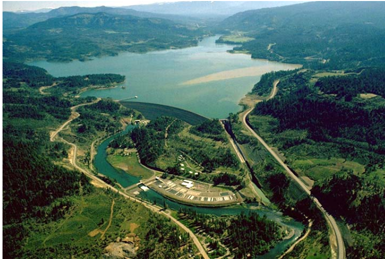
Looking northeast at Lost Creek Lake and the upper watersheds to the east. The Cole M. Rivers Fish Hatchery is below the dam (foreground). Lost Creek flows in from the left and the Rogue flows in from the center back.
